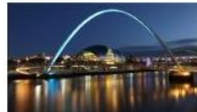
Millenium Bridge Gateshead
